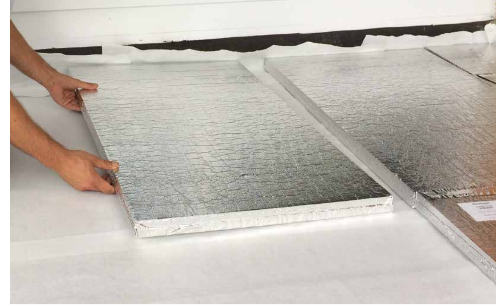
Installation of the Vacuboard for balcony constructions
